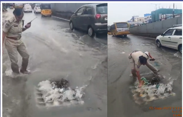
Cop Cleans Clogged Drain
